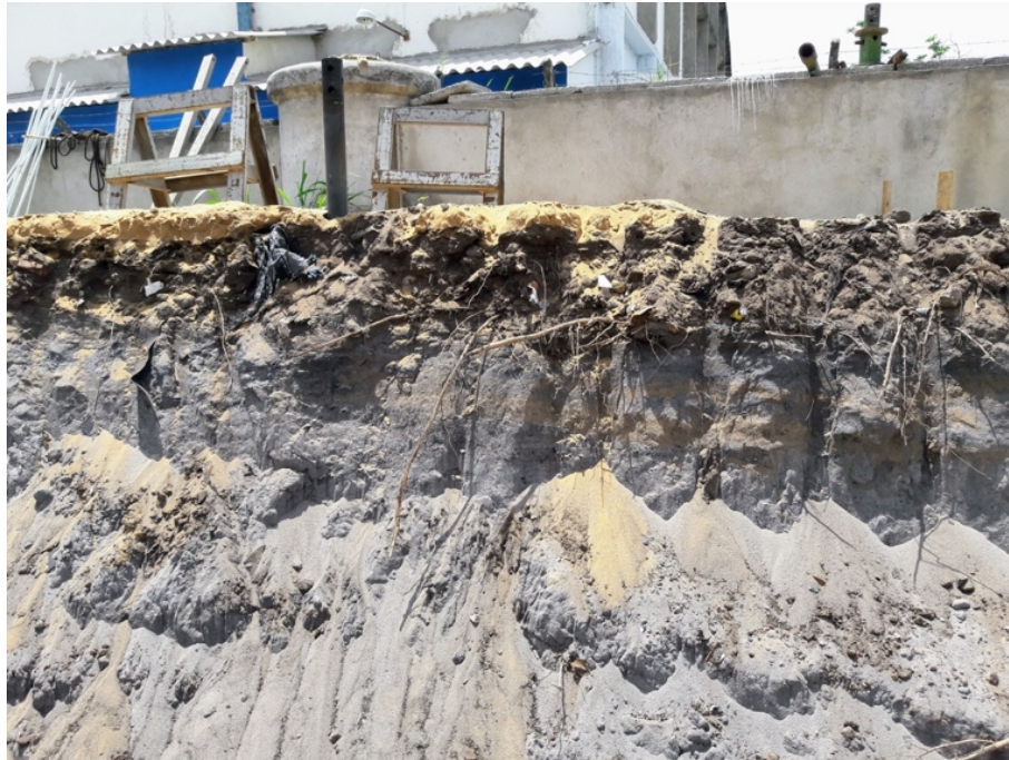
Figure 3.4 – Side view from a cut performed after completion of the pile load testing program.
