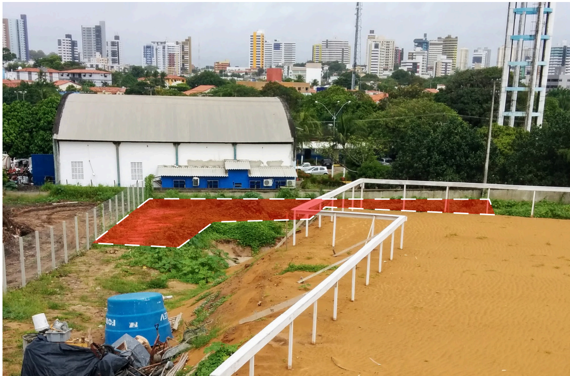
Figure 3.2 – Research site (in red) before the start of construction.
