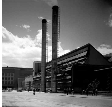
Figura 13 – Dearborn Glass Plant .
