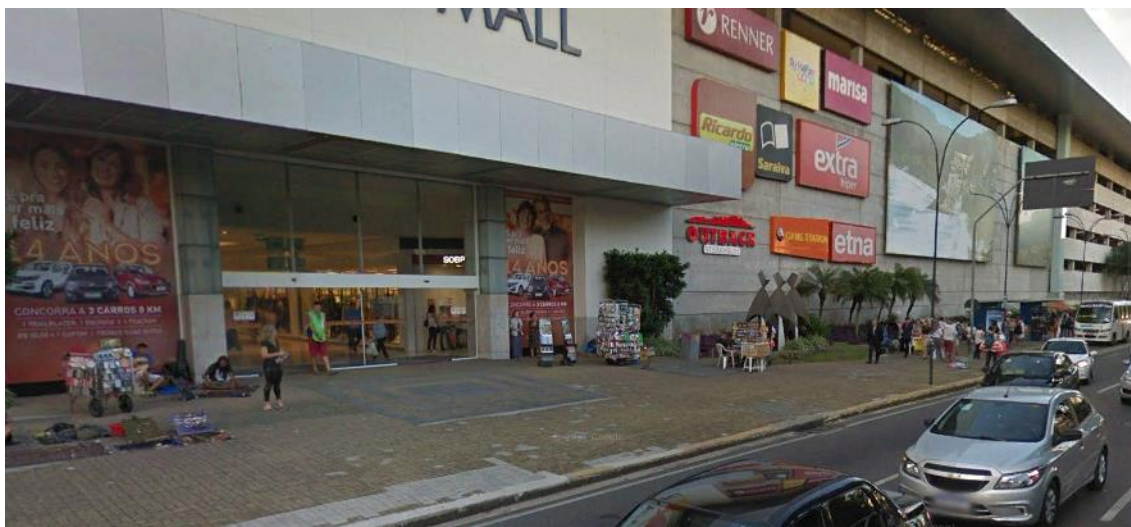
Figura 48: Entrada principal no trecho 02 do shopping Midway Mall.
