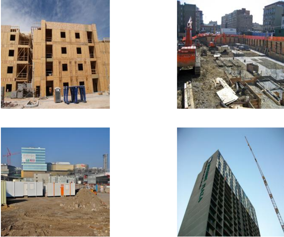
Figure 15 – Gap between images from construction scenario
