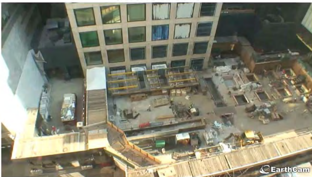
View from 56th Street
