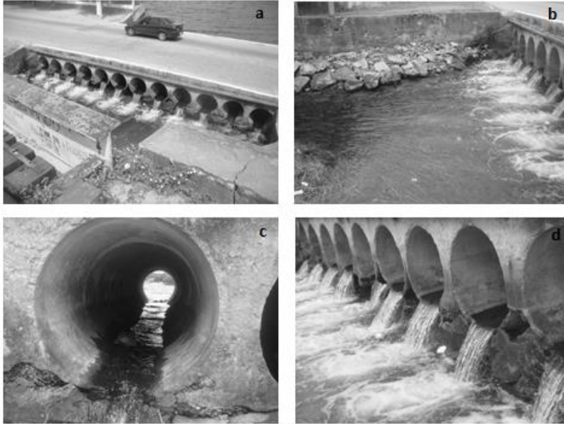
Figure II: a) Bridge that separates Rio Doce and Extremoz Lake b) flow connectivity reduction by rocks (were inserted to avoid siltation procedures) c) low water volume that flows on the crossing-streams d) inadequate crossing-streams which hinder migrations.
